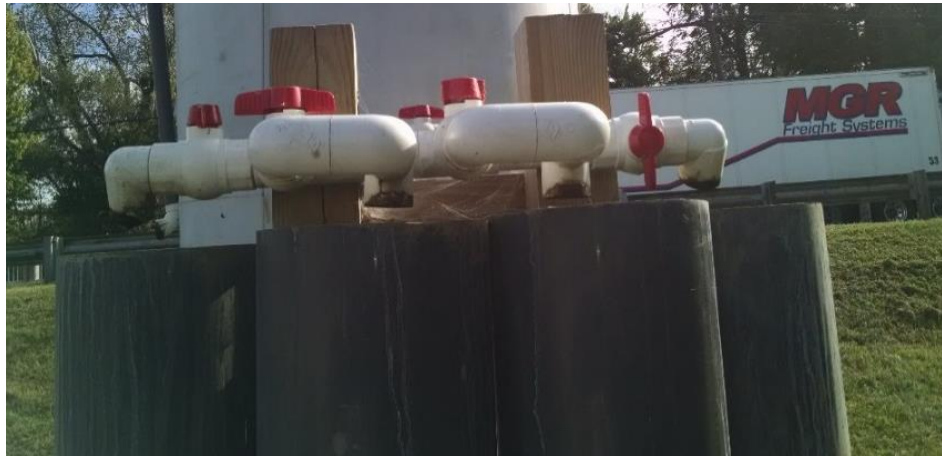
Figure 3.4 Inflow Control into Filters
